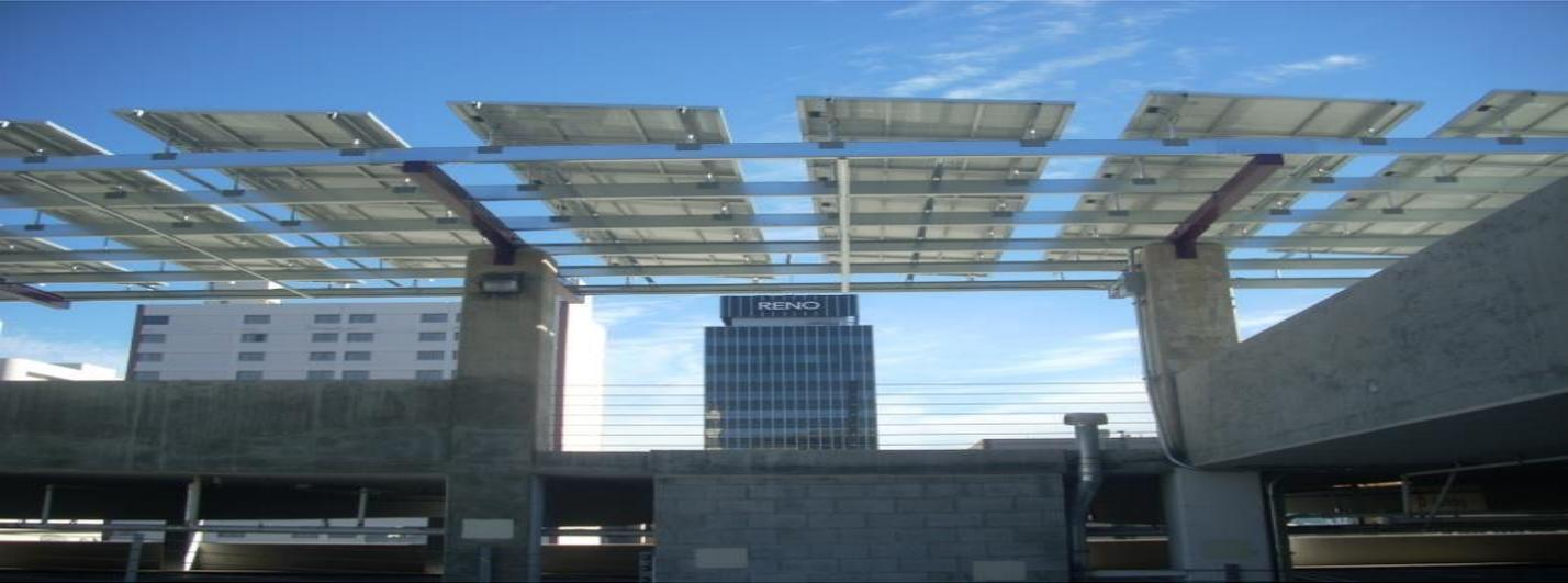
The Reno Event Center Parking Gallery solar PV system consists of 180 Kyocera 205 watt solar modules and one SMA 36 kW grid interactive inverter. The installation strategy adapted an existing steel and concrete parking canopy to accept the racking and modules at a five degree tilt.
